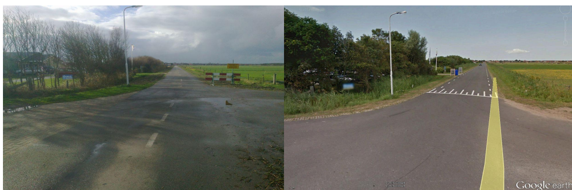
Figure 9: GCP8 during the survey in 2013 (left) and after 2014 (right).
